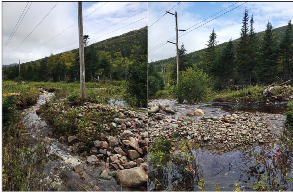
Figure 4: Washout at Structures 453 – TL 226 (left) and 275 – TL 239 (right)
