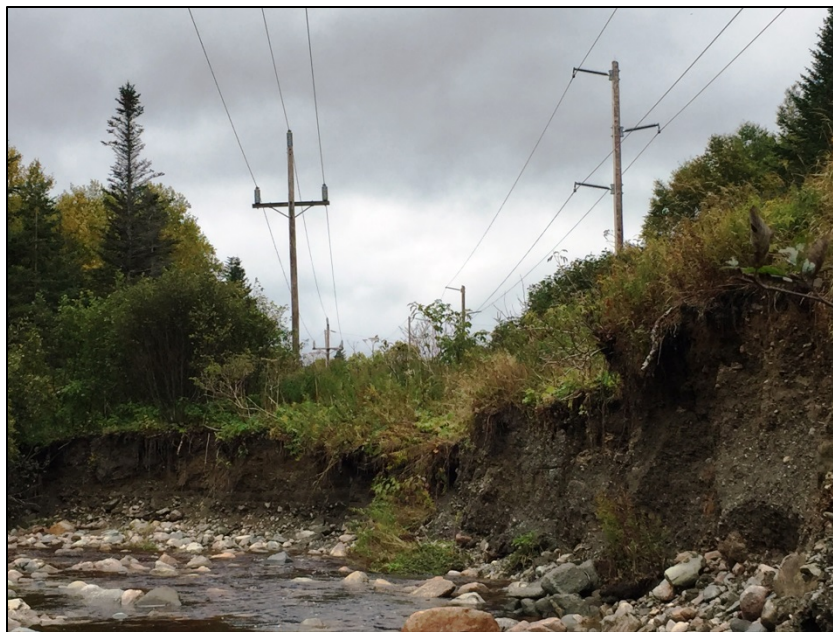
Figure 8: River Erosion East of Structures 278 – TL 239 and 456 – TL 266
