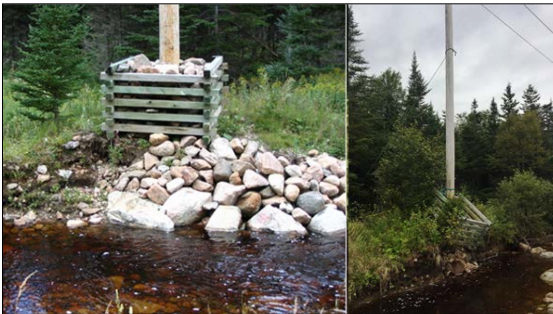
Figure 7: Erosion of Rip Rap at Structure 277 – TL 239 (Circa 2003 on left and September 2018 on right)
